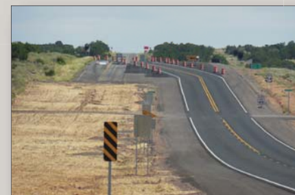
Reconstruction of US 82 will be completed in two phases.
